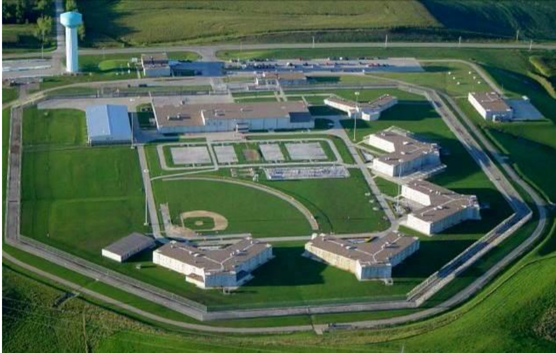
NEWTON CORRECTIONAL FACILITY MEDIUM SITE
