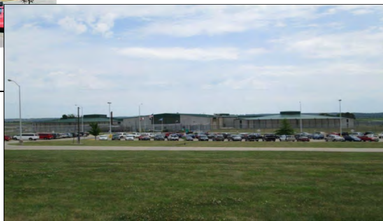
Clarinda Correctional Facility, Clarinda
