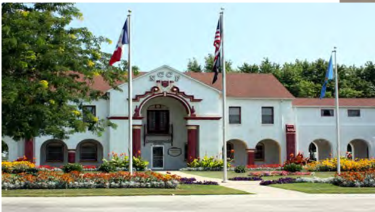
North Central Correctional Facility, Rockwell City
