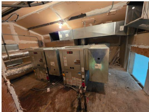
New pump units after installation.
