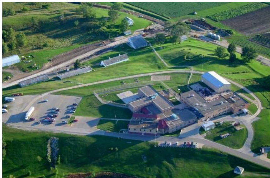
CORRECTIONAL RELEASE CENTER-MINIMUM SITE
