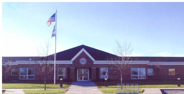
William G. Faches Center • 951 29 th Ave. SW, Cedar Rapids Dedicated in May 20, 1992 The Faches Center houses administrative offices along with pretrial, probation and parole services.
