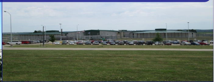
Clarinda Correctional Facility, Clarinda
