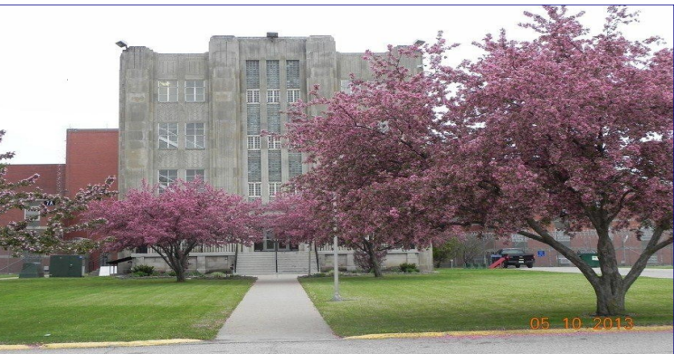
Mt Pleasant Correctional Facility, Mt. Pleasant
