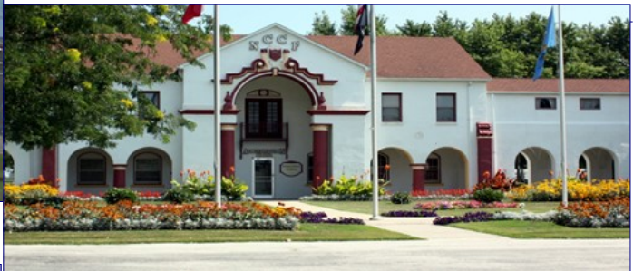
North Central Correctional Facility, Rockwell City
