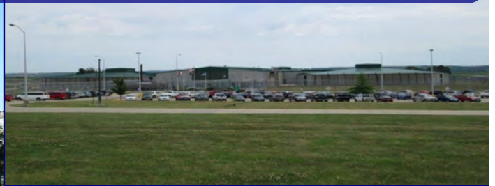
Clarinda Correctional Facility, Clarinda
