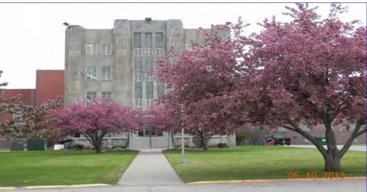
Mt Pleasant Correctional Facility, Mt. Pleasant
