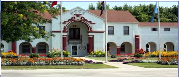
North Central Correctional Facility, Rockwell City
