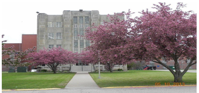
Mt Pleasant Correctional Facility
