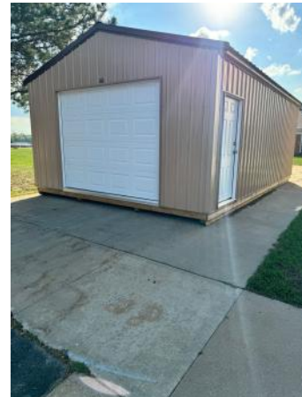
L & C: New drainage tile and groundwater drainage system at Faches Center R: New storage shed at Faches Center
