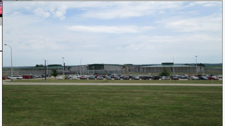
Clarinda Correctional Facility, Clarinda
