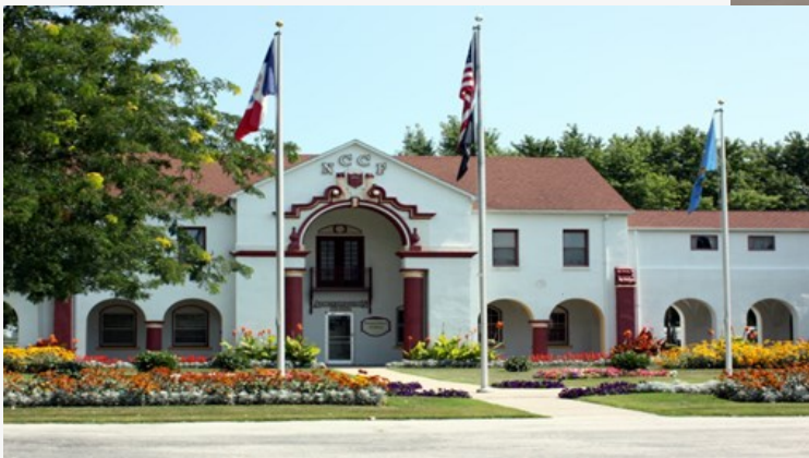
North Central Correctional Facility, Rockwell City
