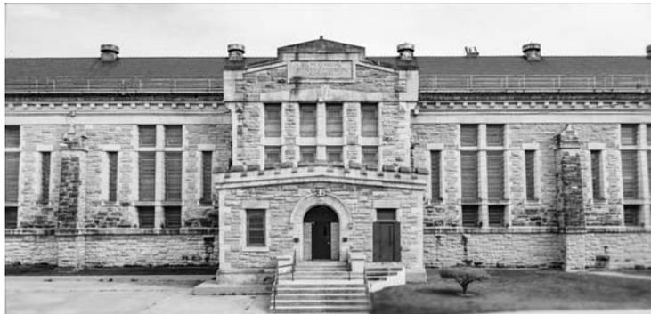
Cell house 218/318 houses general population offenders, encouraging positive adjustment with increased privileges and focusing on programming and release options. It was built between 1910 and 1920 of cut stone masonry and is approximately 33,000 square foot to include 222 cells on five ranges. In 1983, a unitization project was completed at a cost of \$1,311,241 and resulted in the loss of 100 beds.
