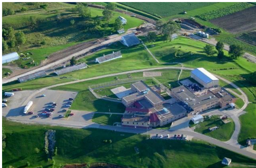
CORRECTIONAL RELEASE CENTER-MINIMUM SITE
