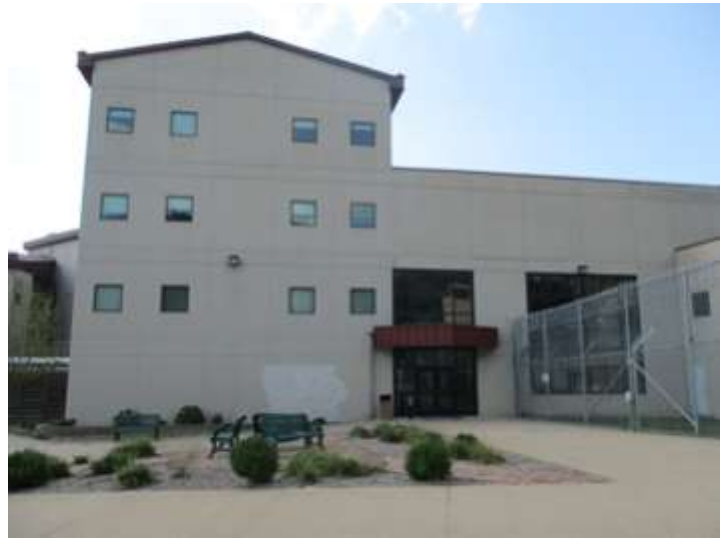
John Bennett Facility Entrance
